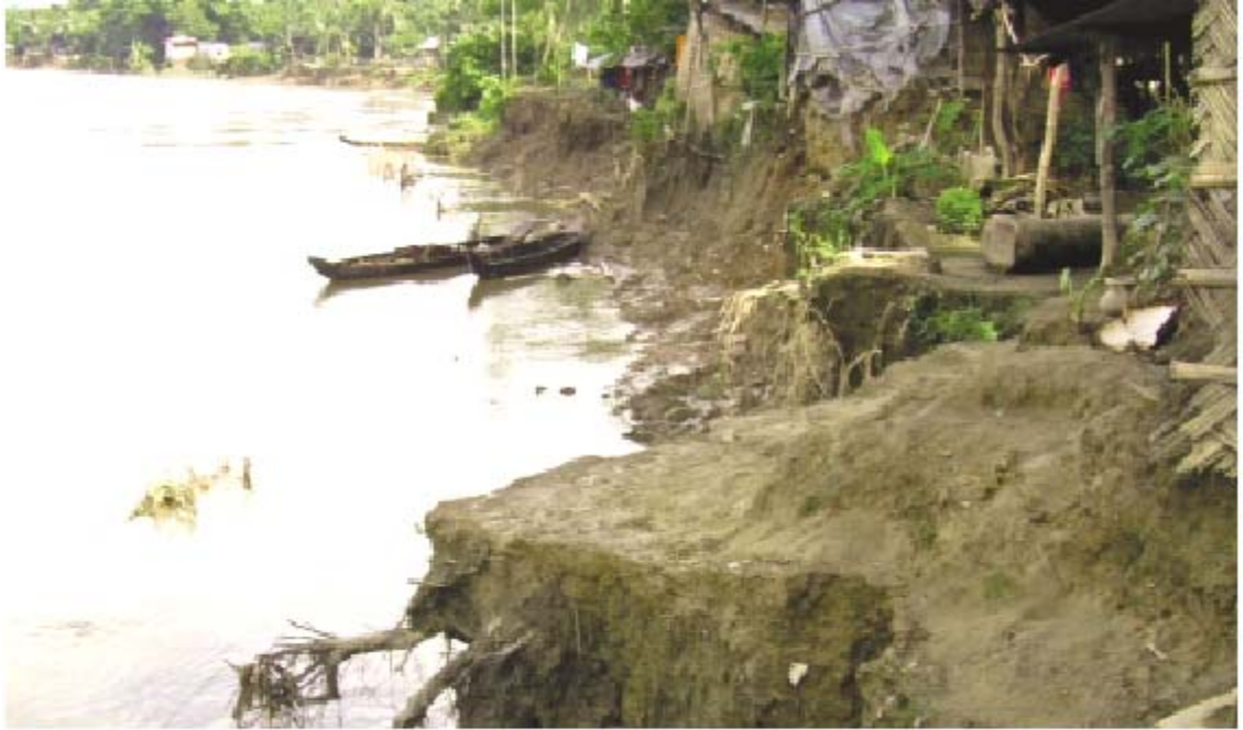
Photo: River bank erosion
